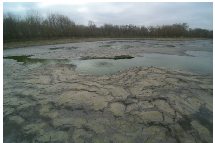
Figure 1: Municipal wastewater lagoon before treatment with Biotifx ® .
