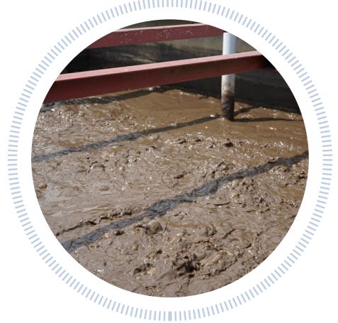
Figure 2. Sludge production was high prior to being treated with Biotifx®.
